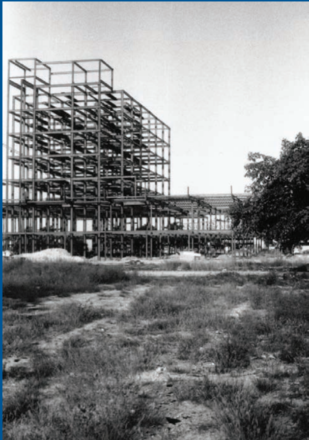
20th Street Terminal under construction - 1957
